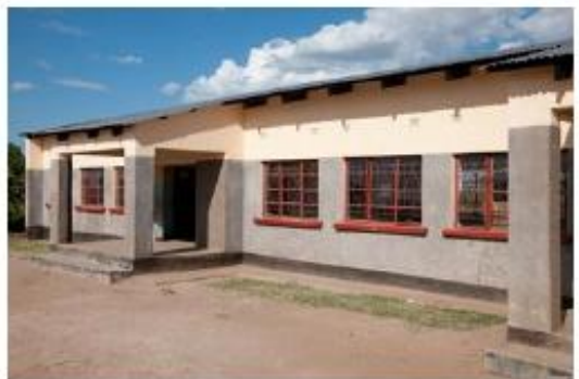
2010: Katapila 1 x 3 classroom block
