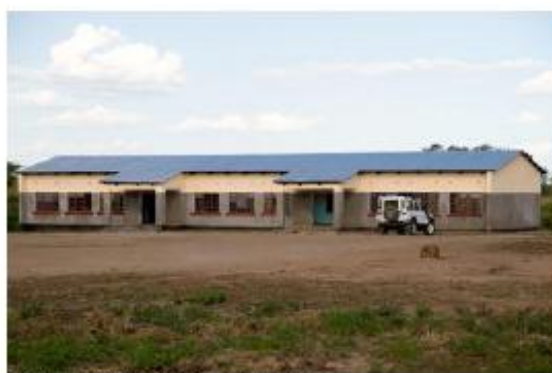
2010: Katapila 1 x 3 classroom block
