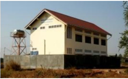
CCH 2 dormitory and skill training centre for sewing and computers.
